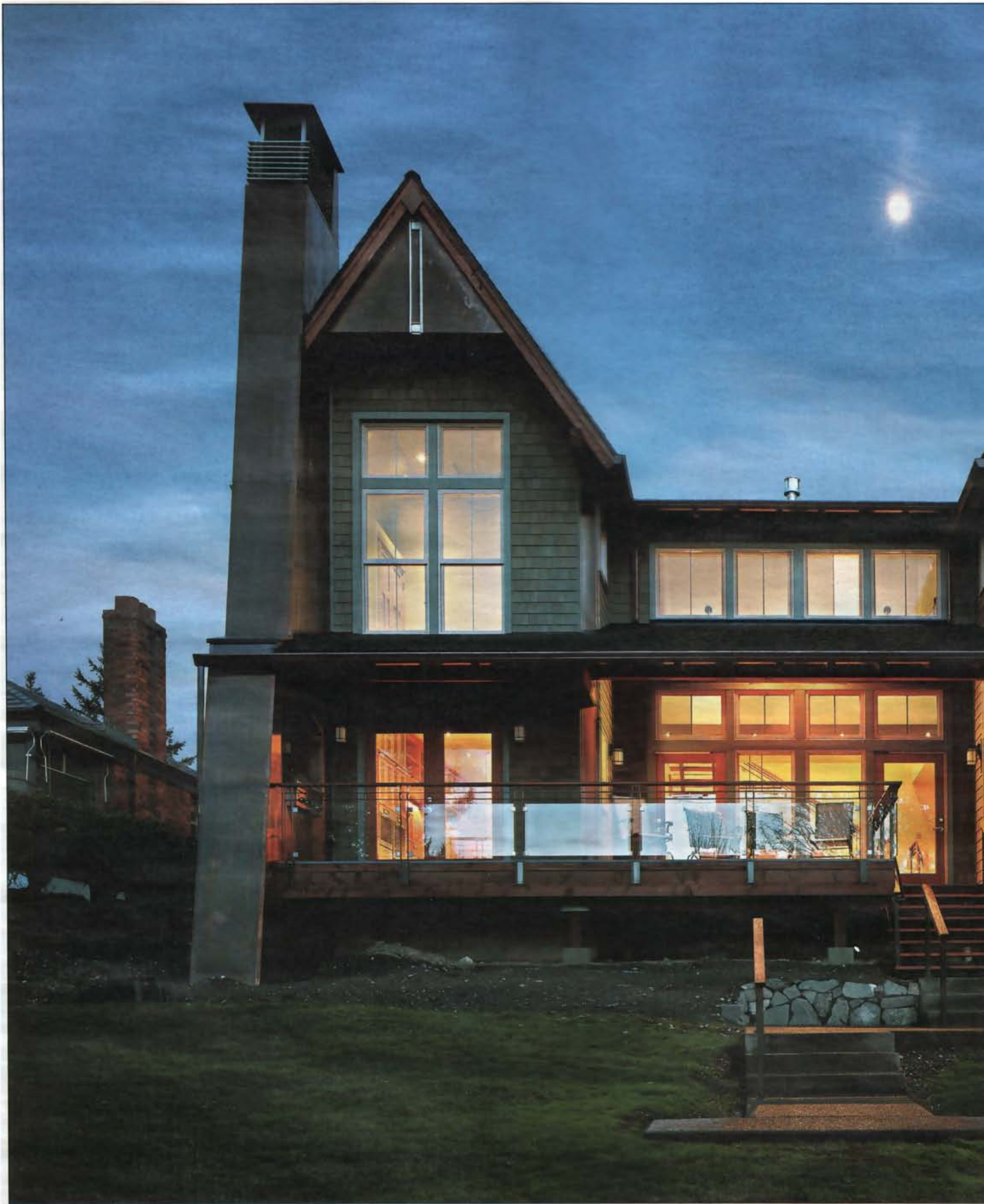
Nancy and Kevin Duffy's new Bernie Baker-designed home in West Seattle seems to float above its site, despite the visual weight of steeply peaked roofs and a copper-clad chimney. Both interior and exterior metalwork is by Steve Johnson of Paracelsus in Port Townsend.
